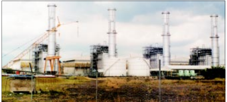
Figure 1. Santa Rita power station viewed from the fuel unloading jetty. Unit 10, the first to complete commissioning is at right of picture. The mobile crane at left is working on preparation of the San Lorenzo site
