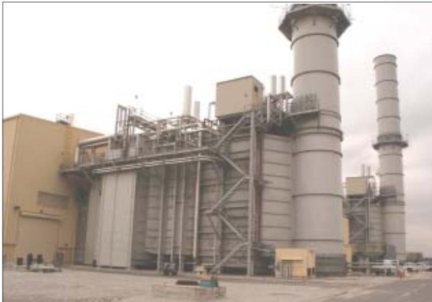
**Fig 4. General view of an HRSG showing sound insulation on the once through section. The yellow hut beside the nearer stack is the emission monitoring position which collects data from both stacks to see that NOx is less than 2 ppm**
