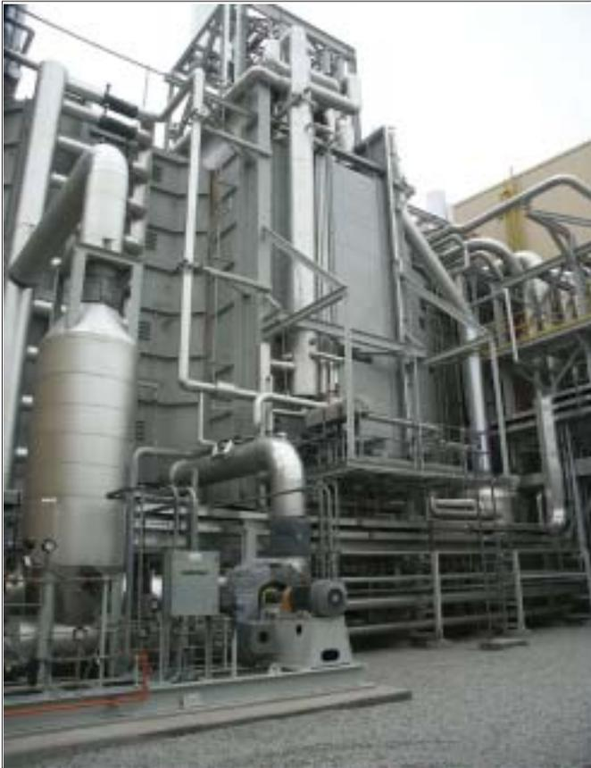
**Fig.1** This view of the HRSG shows the once through section , with heavy sound insulation. The long tube in the centre of the picture is the pressurizer with the blow down tank at left.
