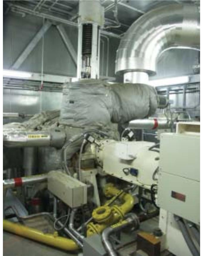
**Fig.2.** The steam turbine HP in its acoustic housing with the 160 bar steam entering from the left. The gearbox, which drops the speed from 8900 to 3600 rev/min, is at right.
