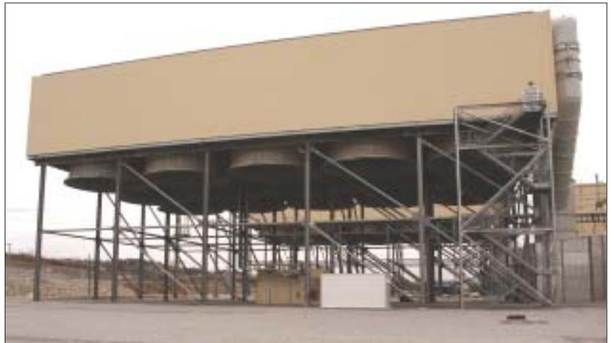
**Fig.6 The air condenser for each block, by Balcke Dürr has 15 cells and is also heavily insulated both in the fan chambers and for the steam pipes, at right of picture, which send the exhaust steam up to the three rows of cooling cells**
