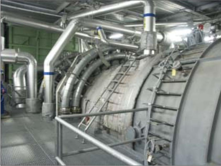
**Fig 3. The gas turbine is housed in a spacious acoustic enclosure shown here looking towards the HRSG with the fuels manifold of the first combustor stage at centre and the cooling air bleed pipes leading off to the OTC units.**
